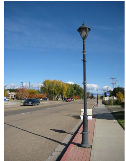
One of Star's sixteen existing decorative streetlights along State Street / Highway 44.
