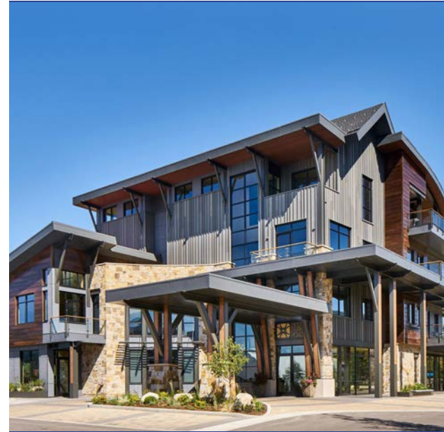
Varying building height and roof treatments
